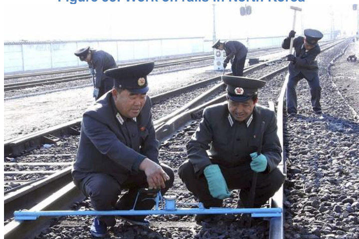
Figure 53: Work on rails in North Korea
