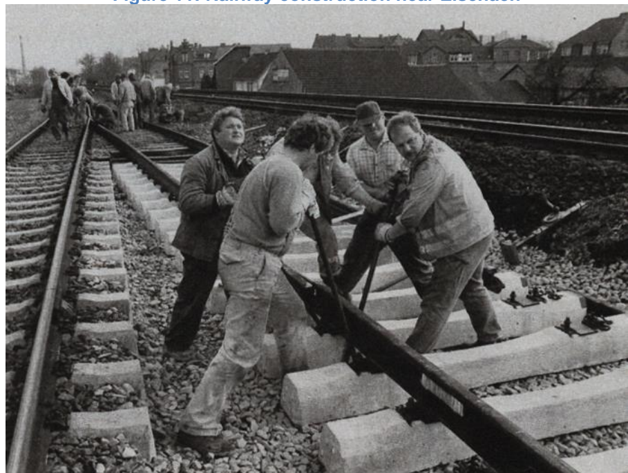
Figure 11: Railway construction near Eisenach
