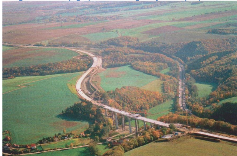
Figure 40: Old (right) and new highway track (left) for A 4
